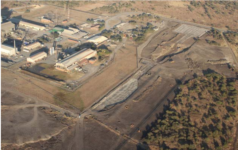
Earthworks - smelter material handling
