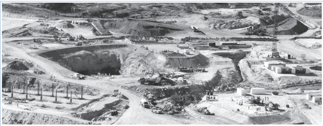
Surface earthworks and the reverse decline boxcut at Booysendal
