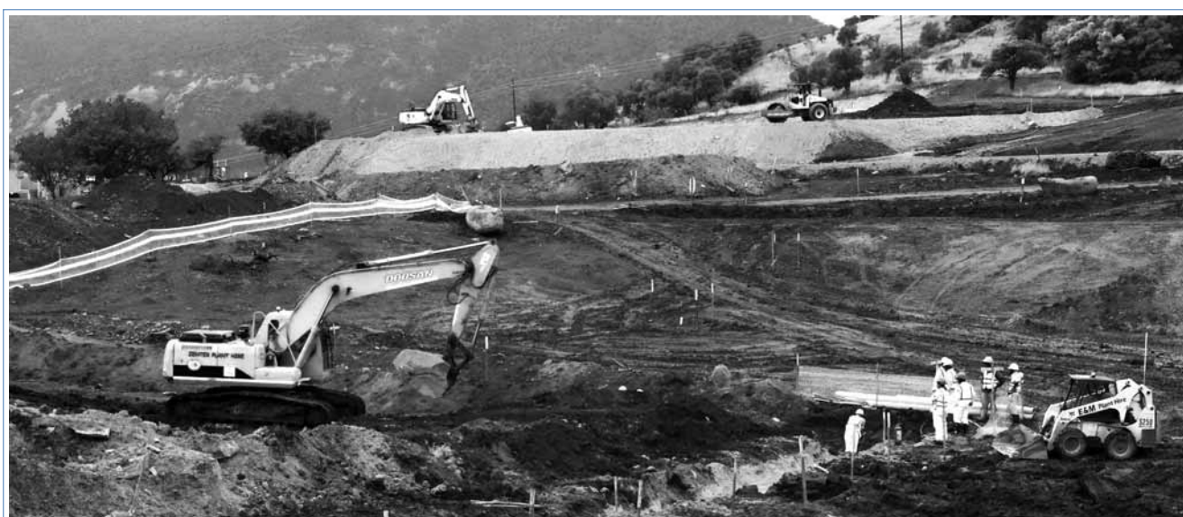
Early earthworks at Booyseindal
