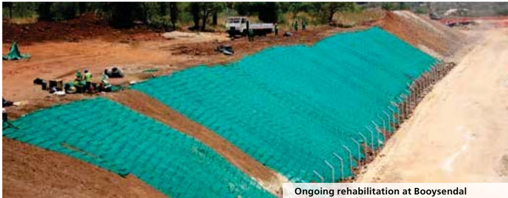
Ongoing rehabilitation at Booyensdal
