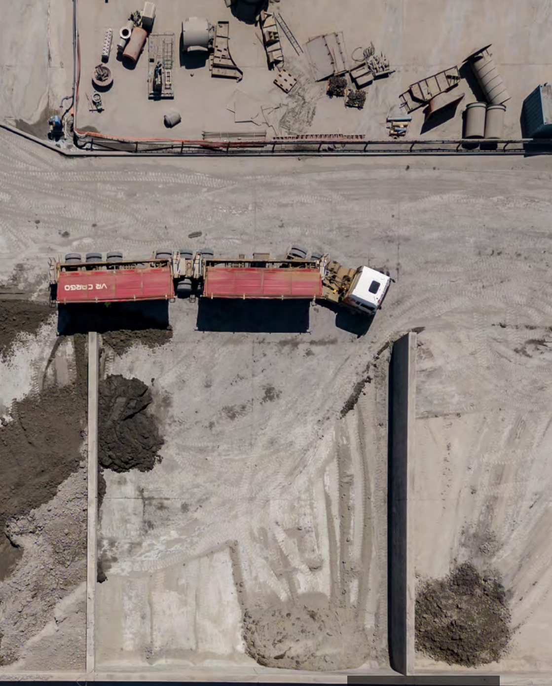
Concentrate storage bays at Zondereinde metallurgical complex
