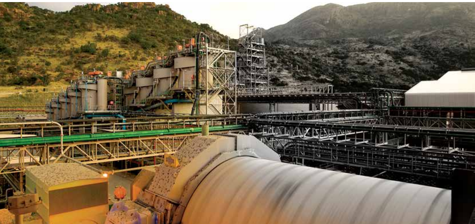
Booyesendal's concentrator plant
