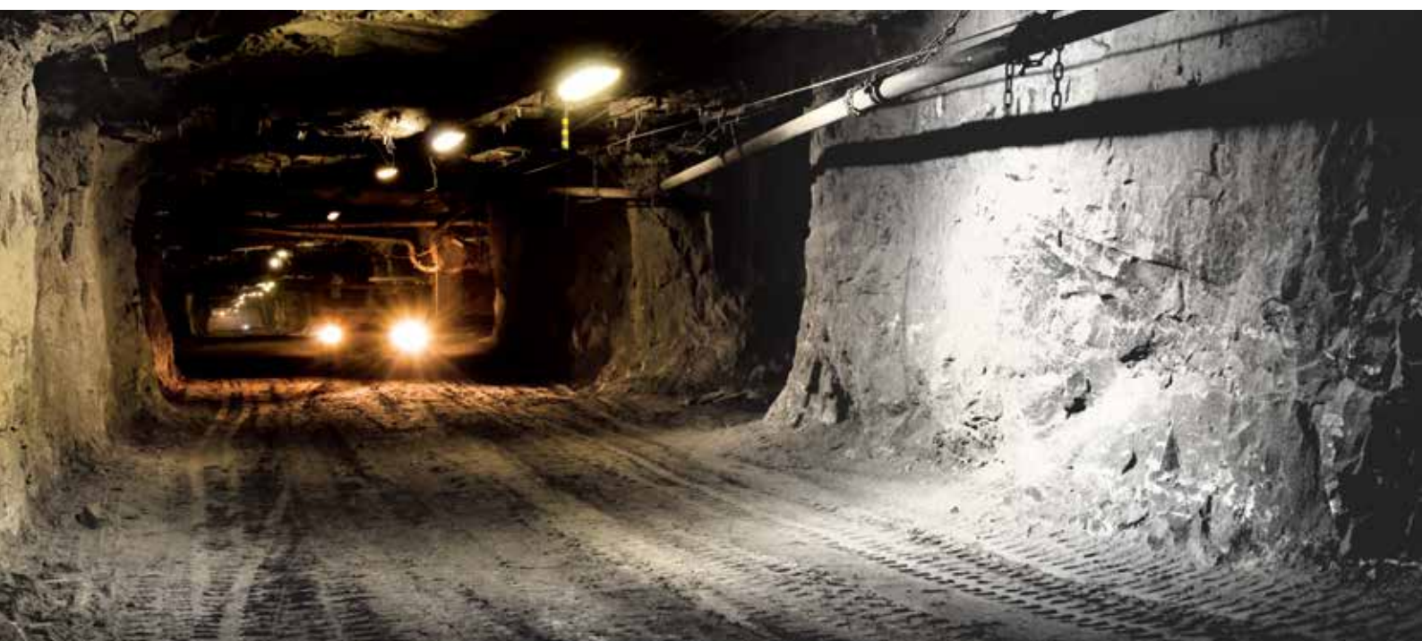
Underground at Booysendal
