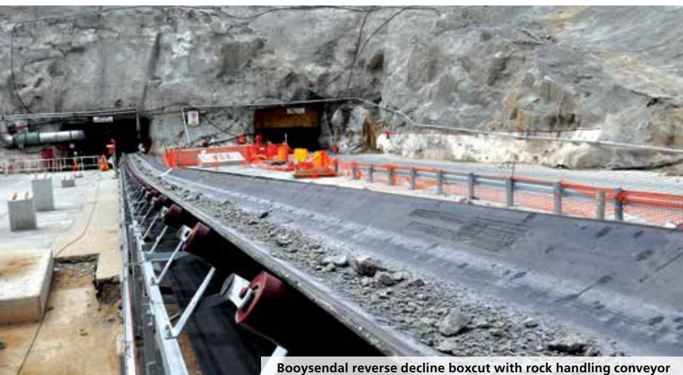
Booysendal reverse decline boxcut with rock handling conveyor
